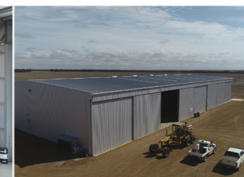
80x30x8.5m with cantilever canopies
